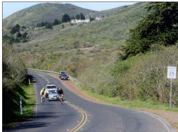
Photo 1.8. Lack of bicycle facilities on Bunker Road.
