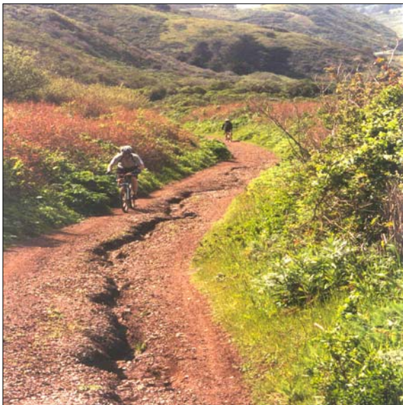
Photo 1.13 Severe trail erosion on Julian Road.
